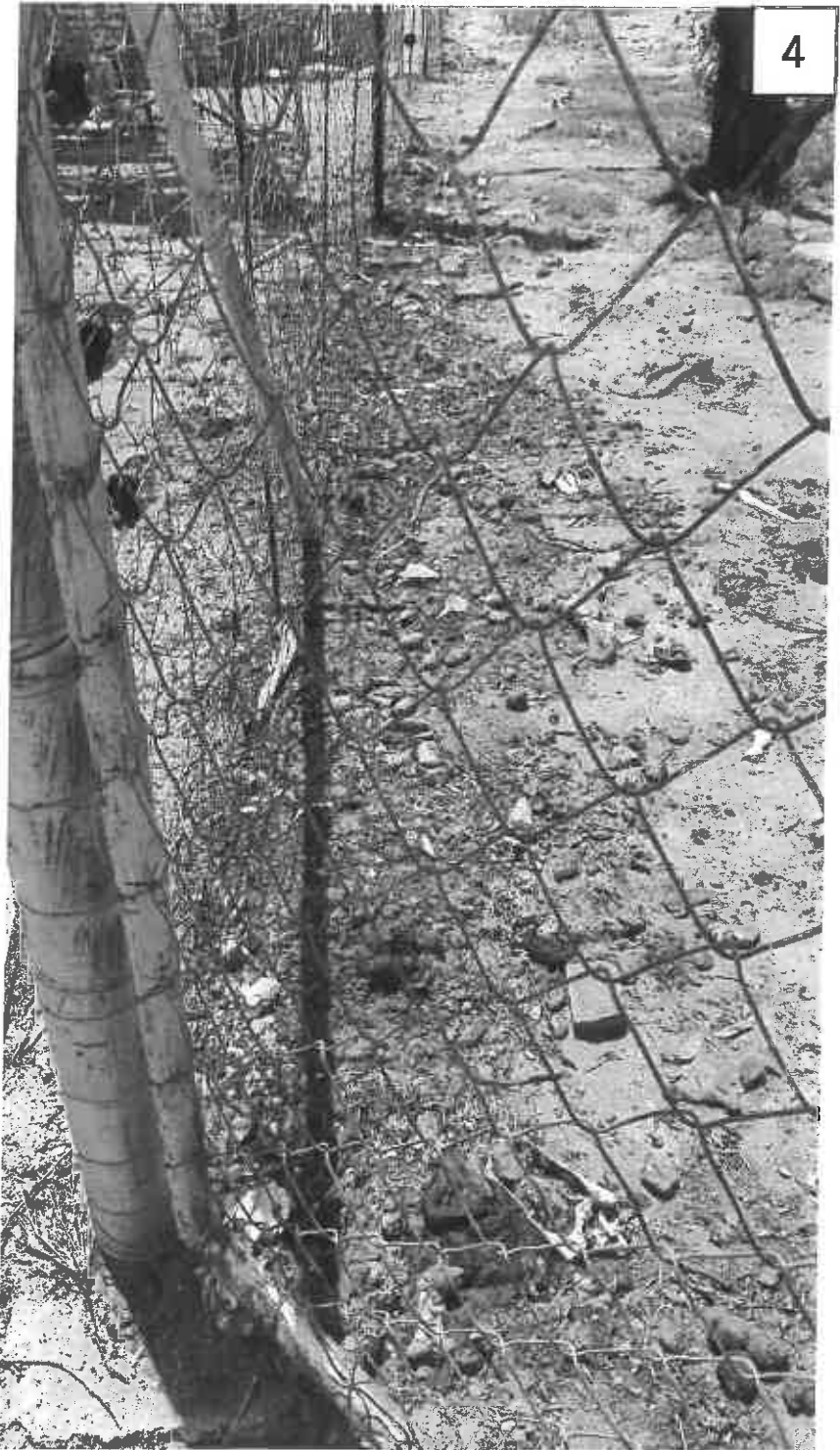
Photo 4 – Vast amounts of accumulated faeces right down the enclosure fence line.
