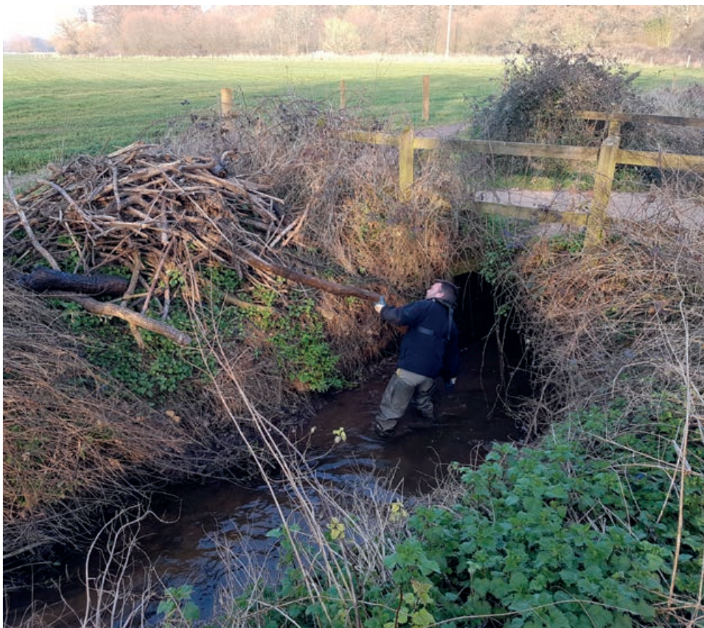
← ROBT Staff clearing a blocked culvert
